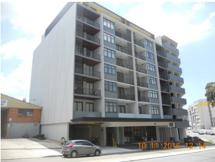
Figure 8 - No. 9-11 Arncliffe Street
