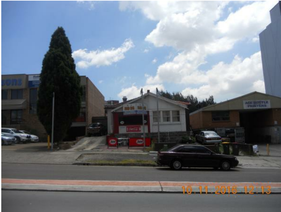
Figure 3 - Subject Site (3-5 Arncliffe Street), and part of adjoining sites No. 1 & No. 7 Arncliffe Street
